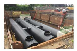
A 120,000-gallon equalization system was installed to substantially reduce combined sewer overflows into the Lackawanna River. This is one of over 60 CSO reduction projects being completed as part of the long-term control plan.
