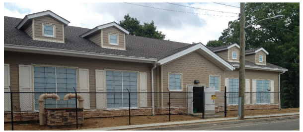
New York American Water owns 10 iron removal treatment plants statewide. The newest one (pictured here) is located in northwest Lynbrook.
