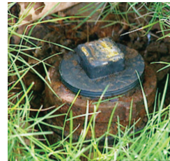
Cleanout sanitary sewer line access
